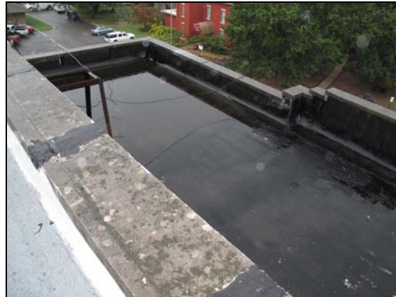
View of north 3 rd floor roof from the upper level.
