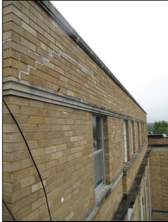
View of minor repairs to the 4 th floor parapet wall.
