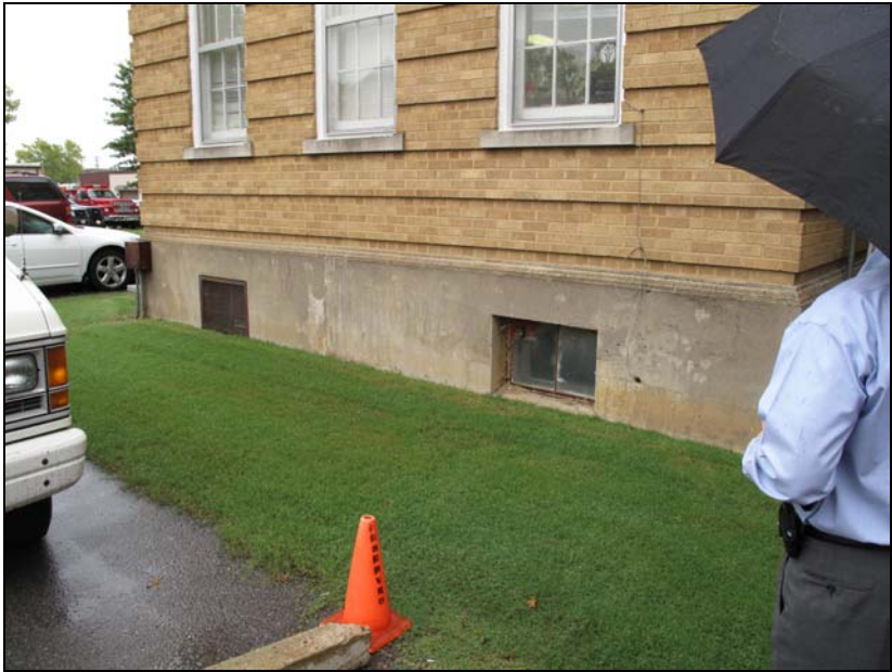
Detail of concrete foundation/basement wall in excellent condition.
