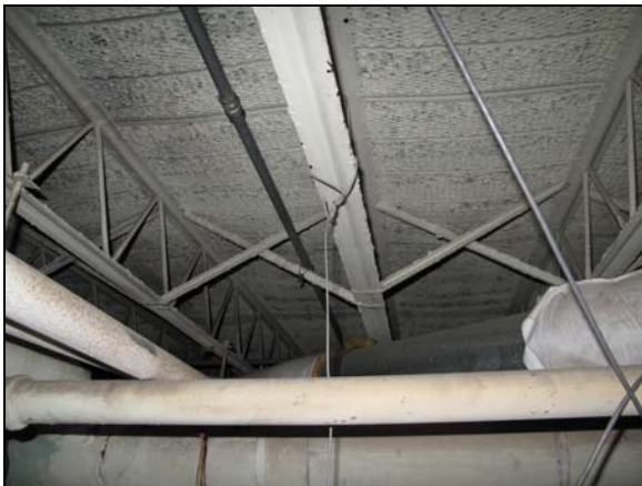
View of the 1 st floor steel and concrete structure.
