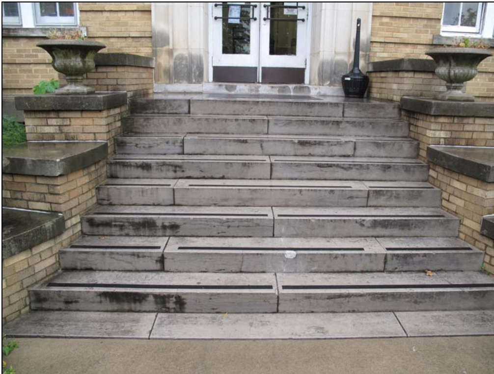
Detail of original limestone steps at east (front) entrance.
