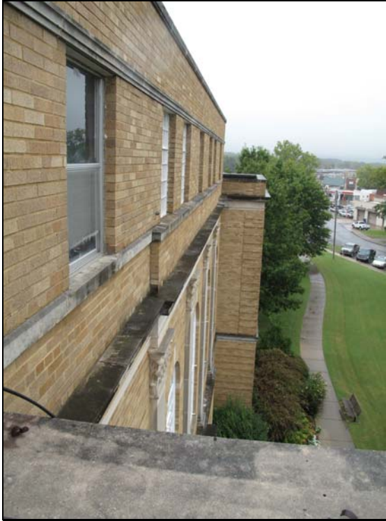
View of east façade from the south 3 rd story roof.
