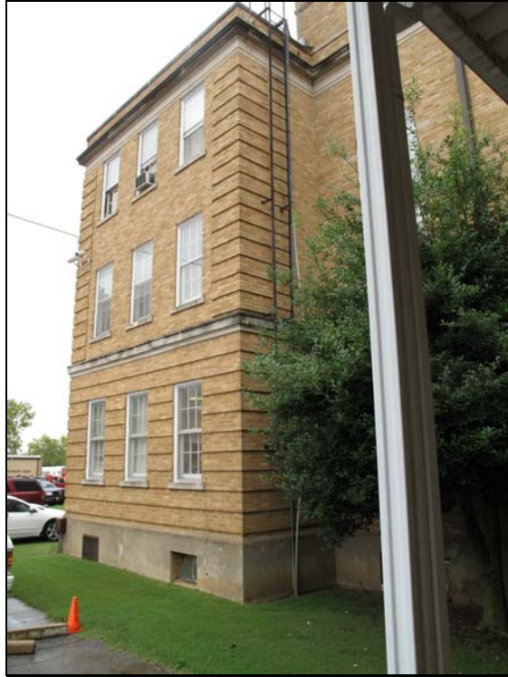
View of north elevation at north corner.
