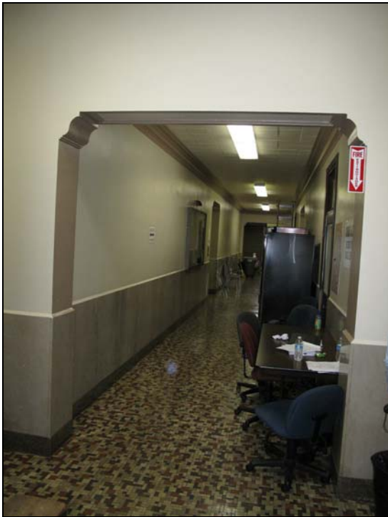
1 st Floor original file, marble wainscot and plaster work.
