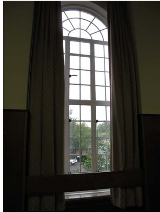
Original steel casement windows
