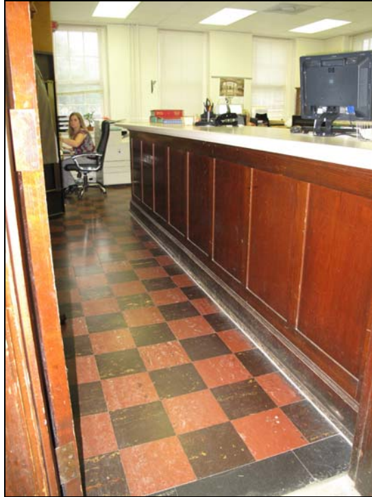
Clerk's office with original VAT floor tile and counter.
