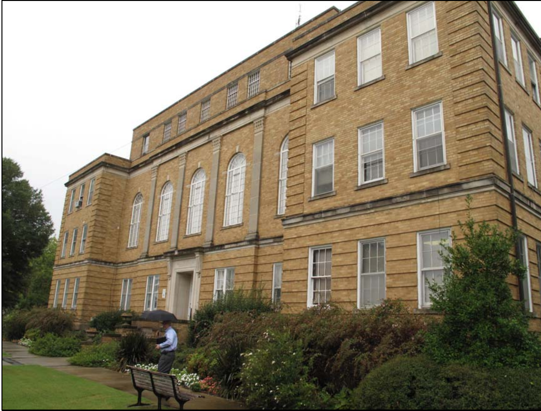
East elevation showing masonry detailing and limestone decorative elements.
