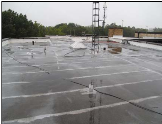
Main roof above the jail looking south.
